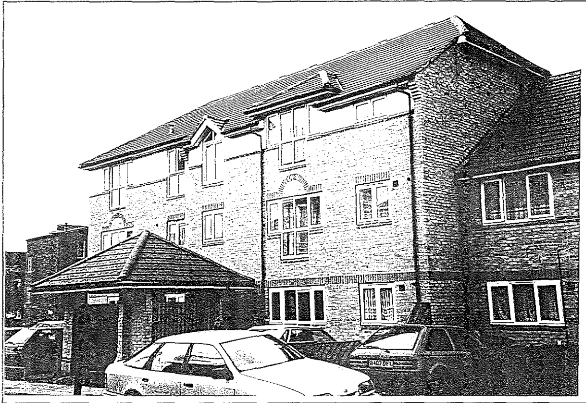
FRONT ELEVATION, 5 JODANE STREET SE8
