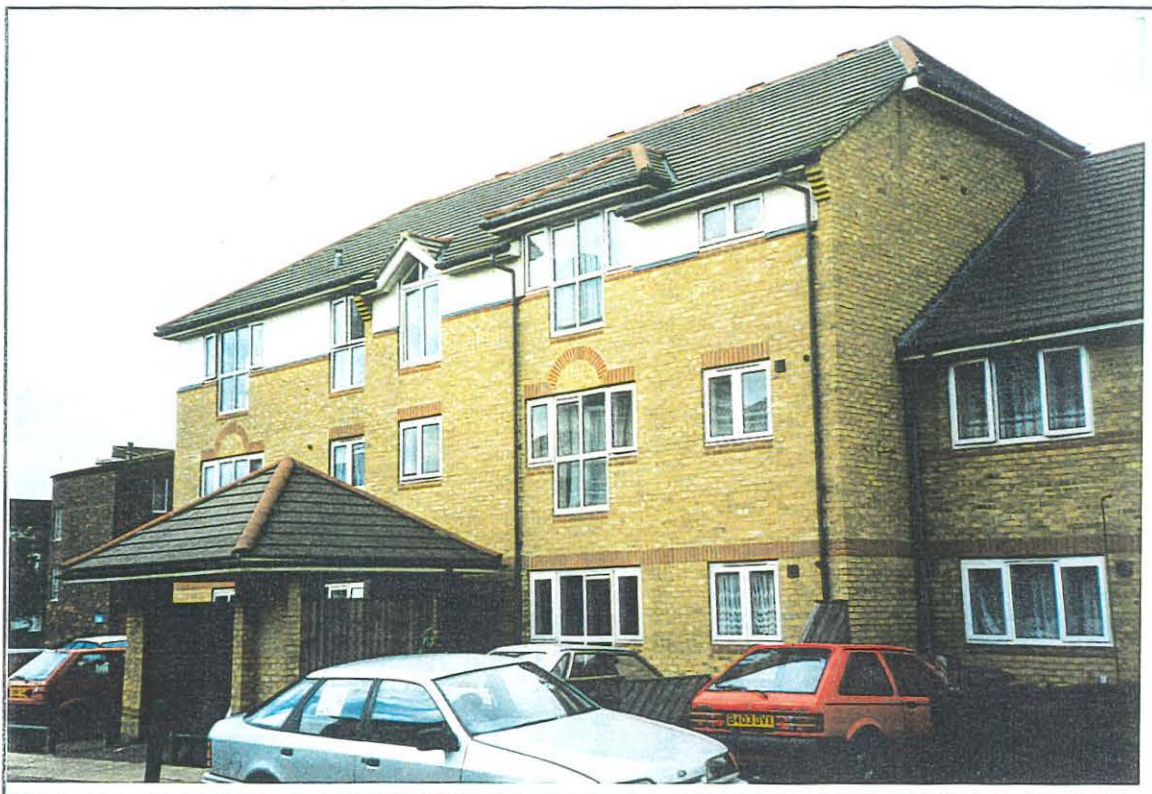
FRONT ELEVATION, 5 JODANE STREET SE8
