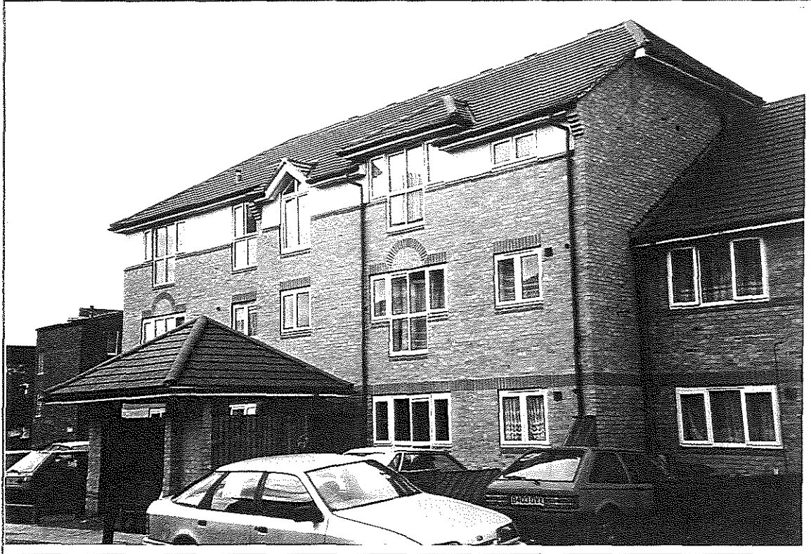
FRONT ELEVATION, 5 JODANE STREET SE8
