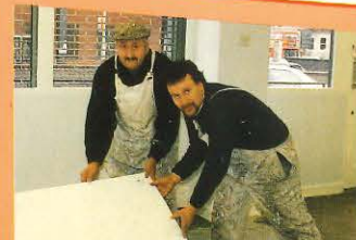
Fitting out an Odeon shop.
