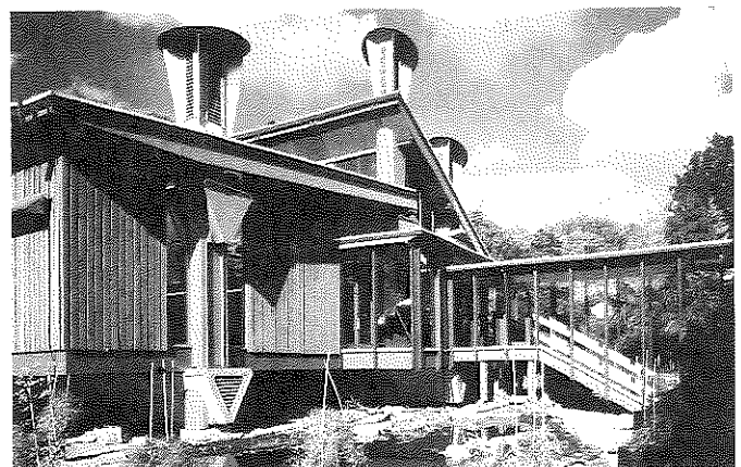
The CUE building: highly commended in the Green Building of the Year Award
